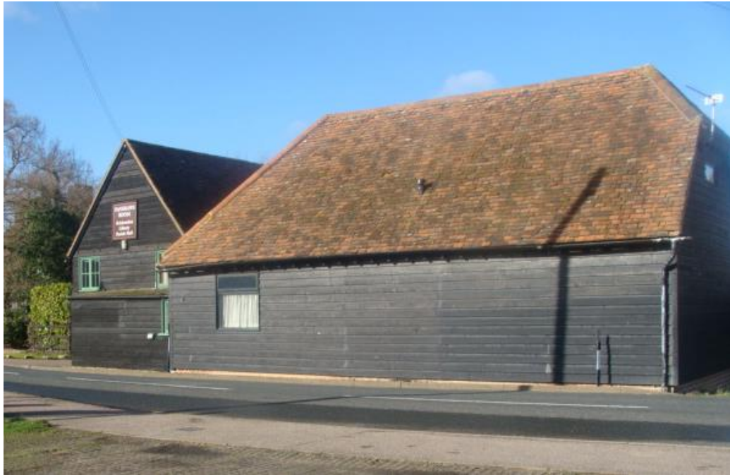
Picture 6 - The village Hall, a successful conversion of to the left - and former agricultural barn. Their success in part has been achieved by limiting the numbers of openings and retaining traditional materials.
