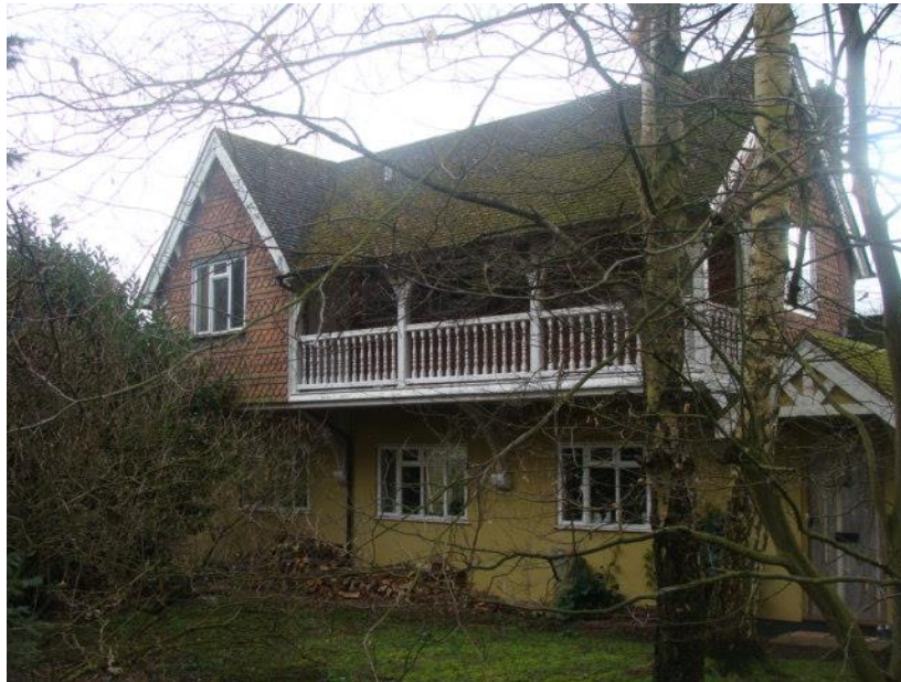
Picture 21. Fieldworker advised this building was a former 'bothy', perhaps used as accommodation for gardening staff to tend nearby greenhouses that once existed in walled garden.
